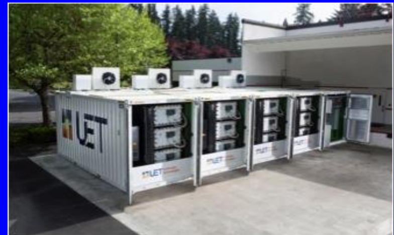
UniEnergy 600 kW/2.2MWh battery system
