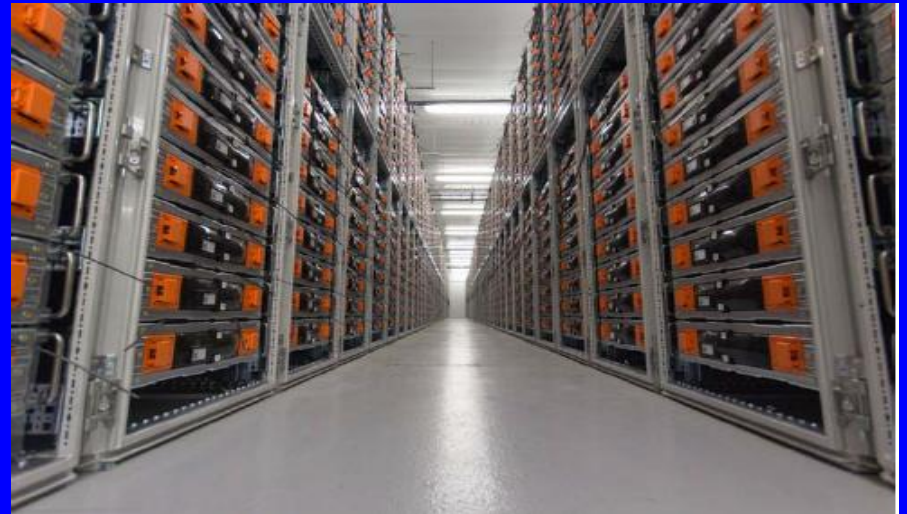
8MW / 32MWh Storage Plant
